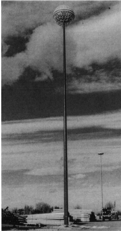
Figure 2. Monotubular light tower.
