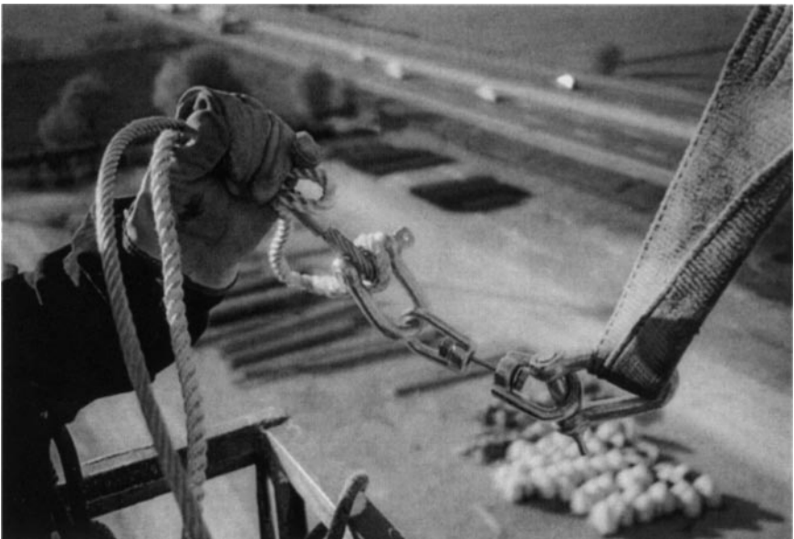
Figure 11. Apparatus for releasing the cable.
